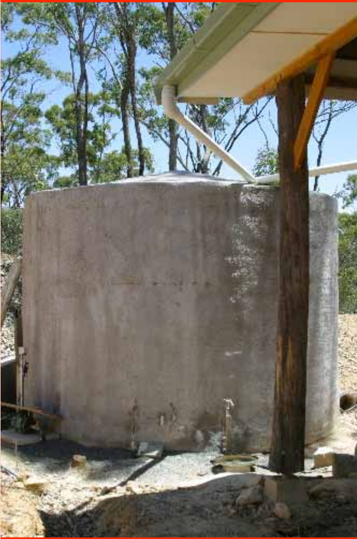
Ferrocement rainwater tank fed from house roof, Fryers Forest Eco-village
